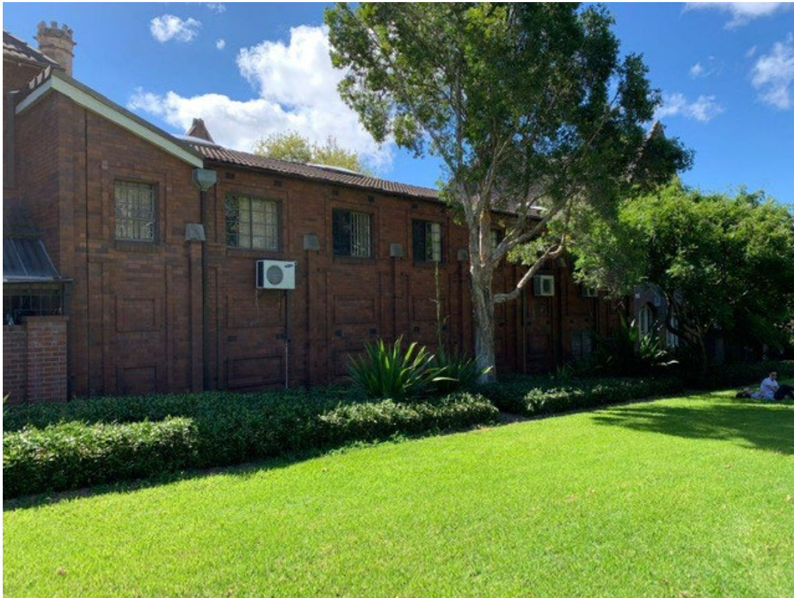
function hall - looking north-west from Prince Alfred Park
