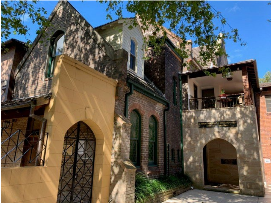
Parish hall - within site, looking north-east
