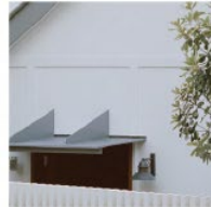
L – CREAM PAINTED FIBRE CEMENT SHEET CANDALEPAS ASSOCIATES – LEE HOUSE
