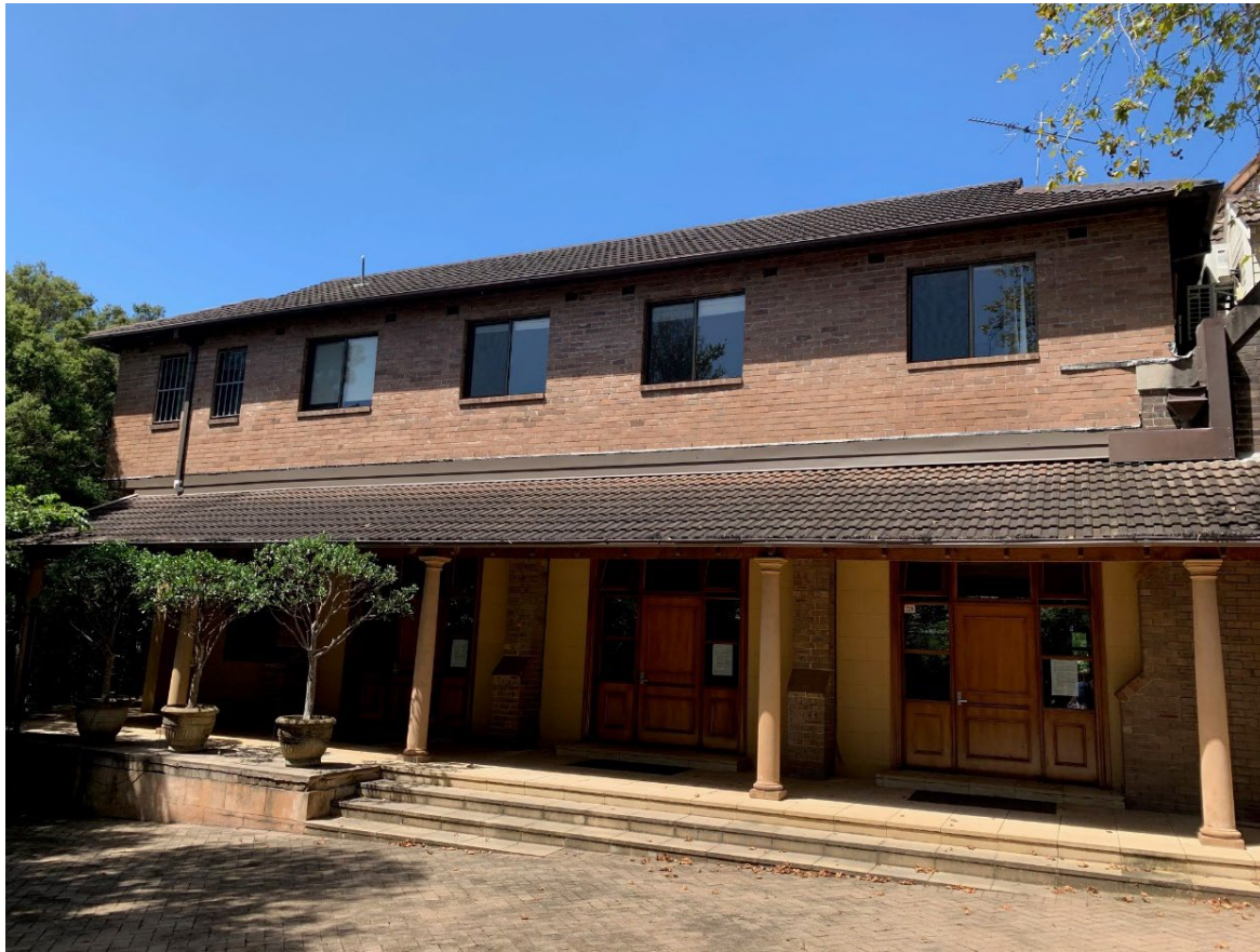
Parish hall extension - within site looking east
