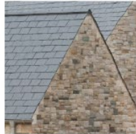
K – SLATE ROOF TILES TERREY HAINES – BLACKSOD BAY
