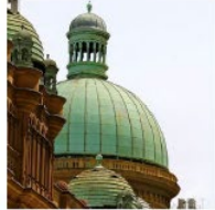
C – COPPER ROOF SHEETING QUEEN VICTORIA BUILDING
