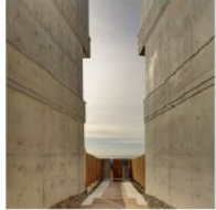
B – OFF-FORM CONCRETE CANDALEPAS ASSOCIATES – PRINCE STREET CRONULLA
