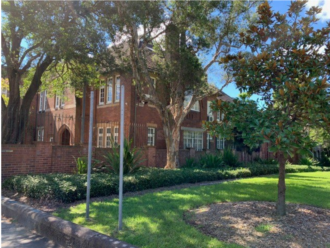
former St Paul's Rectory - looking north-west from Cleveland Street
